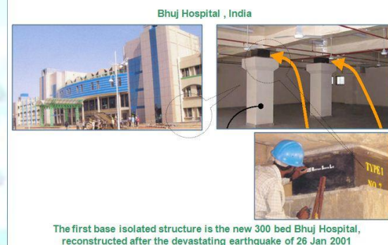
Fig.7: Hospital at bhuj, India retrofitted with Base Isolators.
